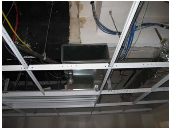
Photo 4: Unprotected duct opening
