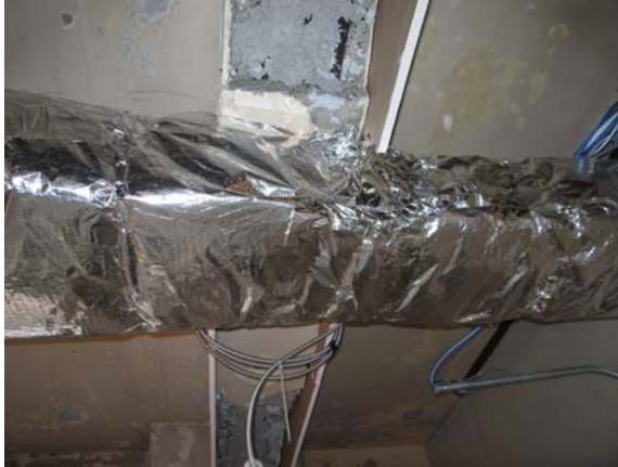
Photo 1: Un-insulated top of duct
