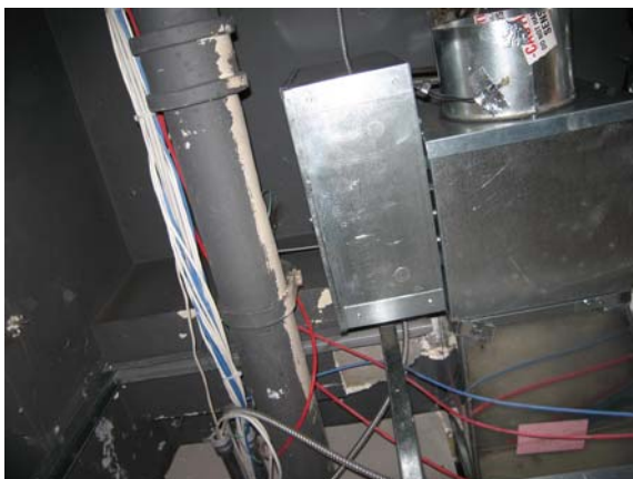
Photo 3: Inaccessible VAV Controls
