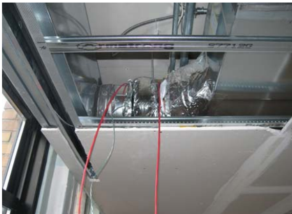
Photo 2: Un-insulated Linear Collar
