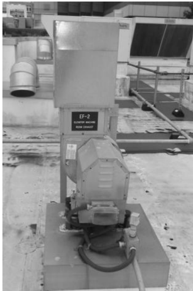
Figure 2.2: EF-2 Elevator Machine Room
