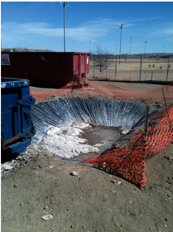
Concrete washout
