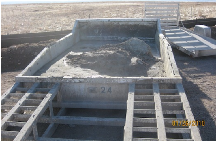
Concrete washout
