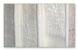
the occupants by an approved thermal barrier of ½" thick (12.7 mm) gypsum wall-board or an equivalent 15-minute thermal barrier complying with, and installed in accordance with, IBC Section 2603.4, IRC Section 314.4 or UBC Section 2602.4, as applicable, except when installed in attics and crawl spaces. Maximum thickness of the insulation is 6.5" (165 mm) in the walls and 9.5" (241 mm) in the ceiling.
