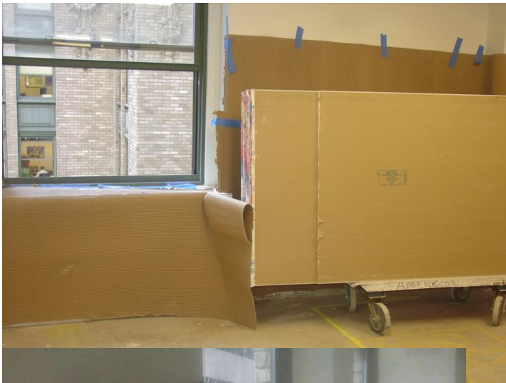
12/5/2008 SMACNA 3.3.6 Cover – Seal Existing exhausts were covered.
