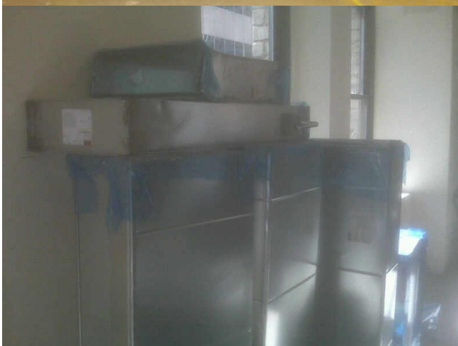
5/27/2008 SMACNA 3.1 HVAC Protection Duct openings were covered once unwrapped and stored on site.
