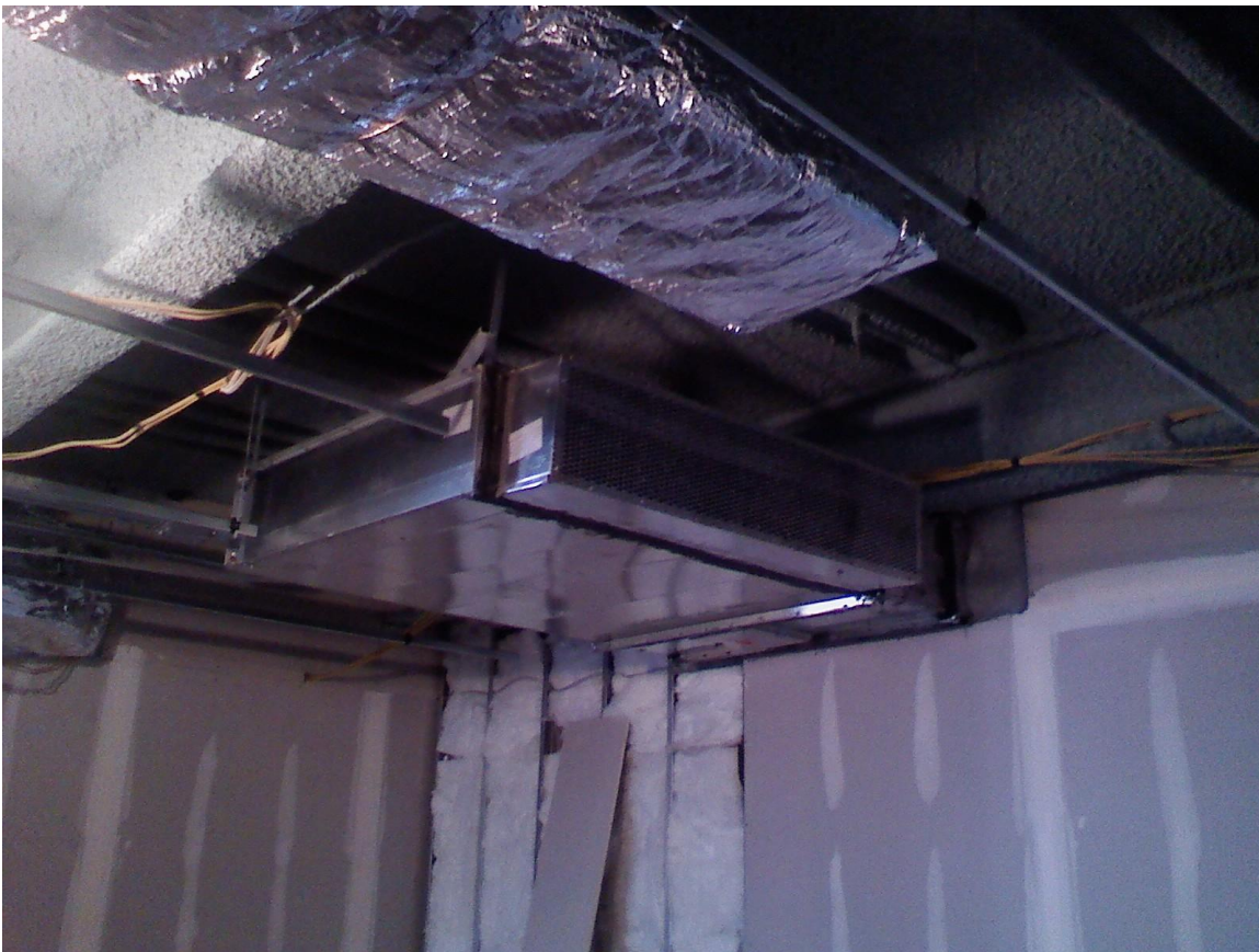
Building Return-Air Duct sealed off during construction process.
