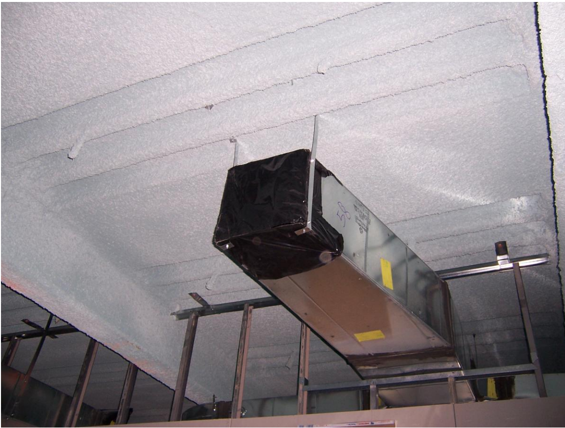
All new duct work was sealed until connection.
