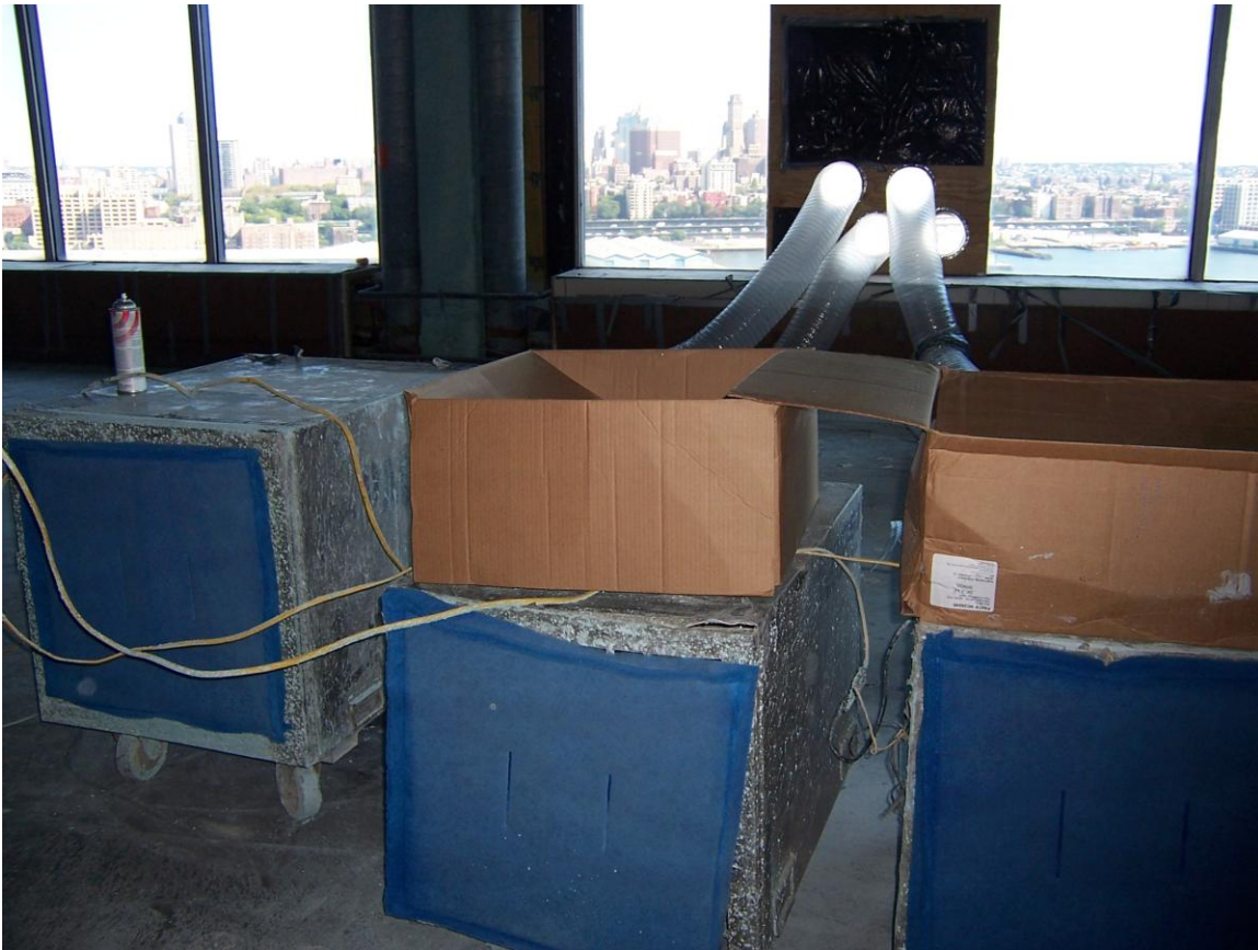
Micro Traps Located on Floor Thru-out 75% of Construction phase. Filters were changed regularly.
