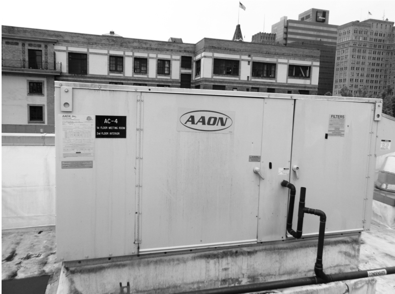
Figure 2.2: Typical Roof Top Packaged AC Unit
