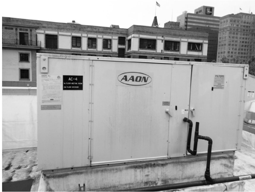
Figure 2-2: Typical Roof Top Packaged AC Unit
