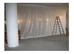
Typical plastic curtain wall to contain dust during construction.
