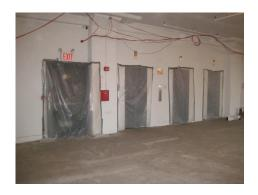
Base building elevator bank was sealed to protect shaftway from construction/demolition dust.
