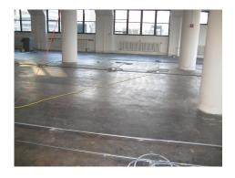
Sealed concrete floor to reduce airborne elements in under floor plenum.
