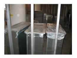
Sealed duct work delivered to site before installation.
