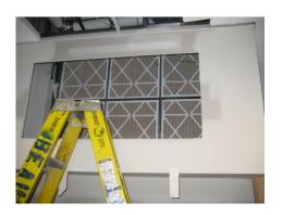
MERV 8 filters installed prior to unit start up
