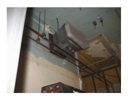
Base building duct sealed prior to work beginning.
