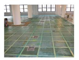
Sealed raised floor prior to carpet installation to maintain dust-free conditions
