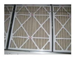
Typical MERV 8 filters used for initial start up of the system. Filters to be upgraded to MERV 14 prior to occupancy
