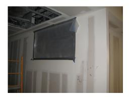
Sealed return air duct that supplies typical air handling unit prior to unit start up
