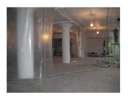
Typical plastic curtain for column work to control dust while columns were being refinished.
