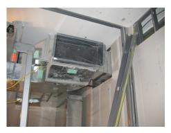
Installed duct work with seal intact until final connections could be made.
