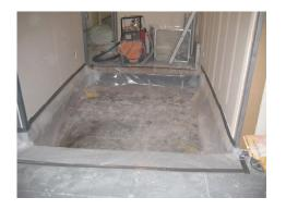
Temporary sealing of raised floor where new air handling unit will be installed. This is to protect under floor plenum before air handling units could be installed.
